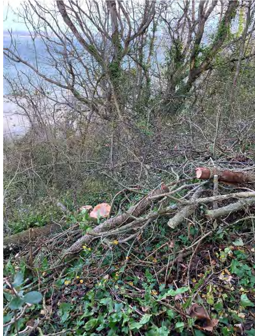
Line 65 IOW_5_S062 to 68/ Tree Works (1)
