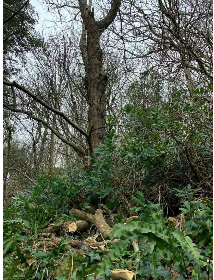
Line 52 IOW_4_S026 to S028/Tree Works
