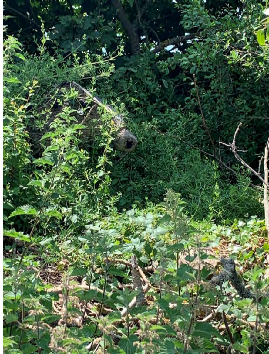
Line 51 IOW_4_S023 to S025/ Tree Works (1)
