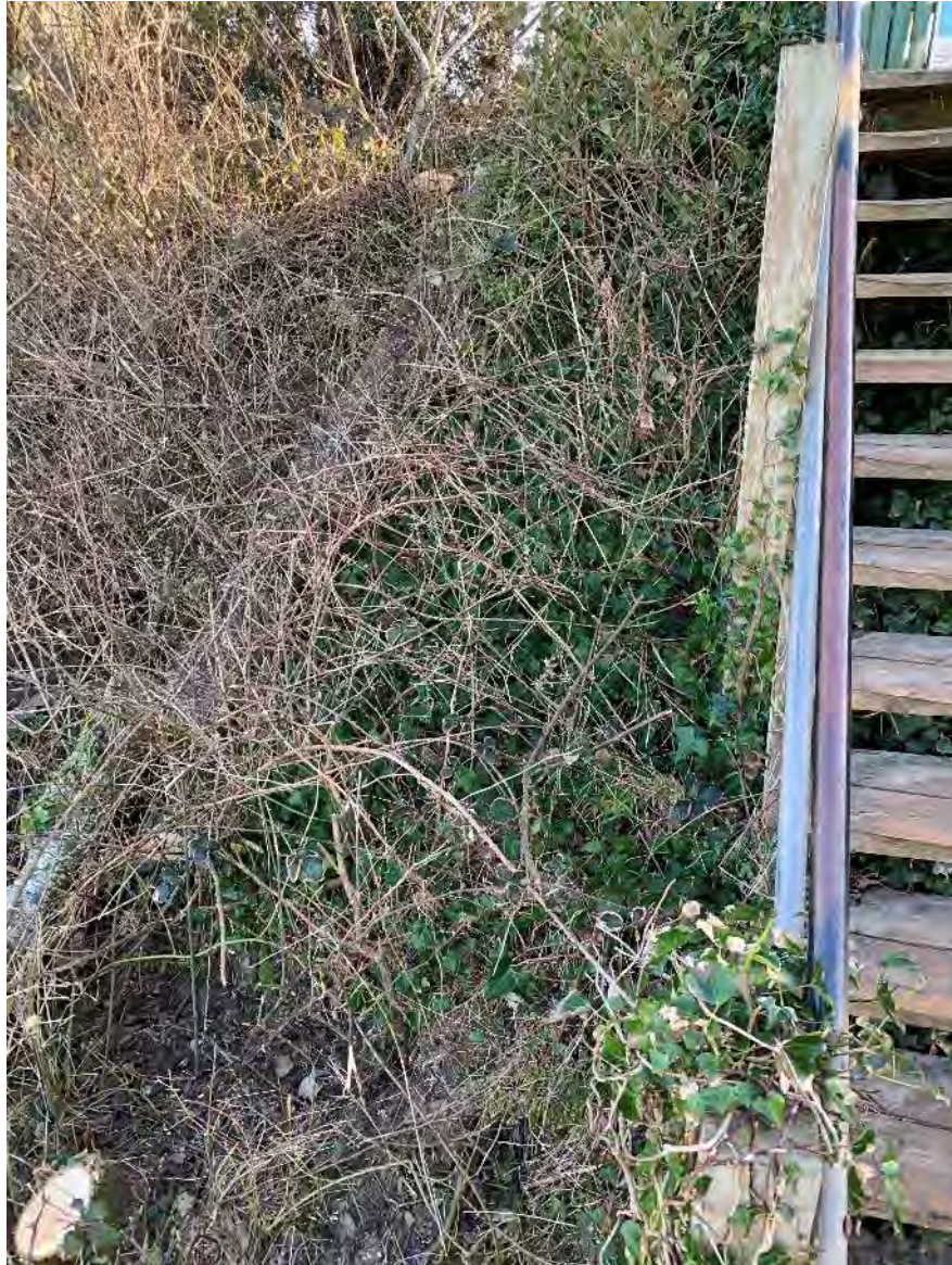
Line 64 IOW_5_S054 to 59/Tree Works (2)
